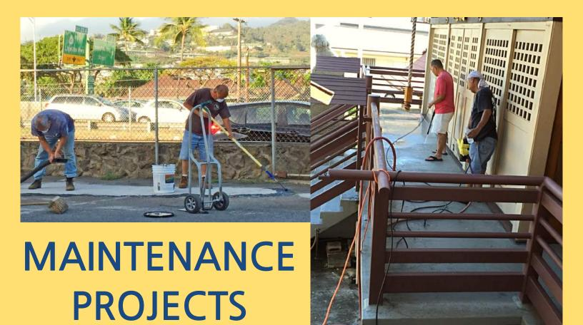
The Pothole Blitz continues with application of a seal coat to fill minor surface voids and protect the surface from water penetration, oils and UV damage.
