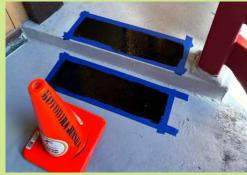
The old non-skid safety strips in front of the shrine door were removed. Glue seeps into concrete pores which made removal a challenge. A non-skid paint with carborundum aggregate was used instead of the strips.
