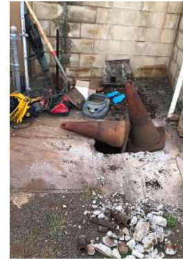
Concrete removed to expose old valve
