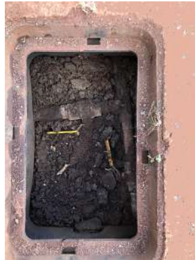
Shrine's main valve covered in dirt and debris
