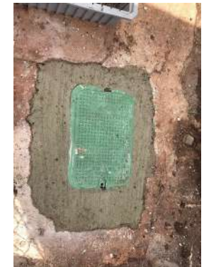
Concrete laid after replacement and repairs completed
