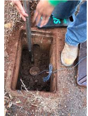
BWS crew removed dirt and shut off the valve
