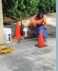
edge of the cracks. He then coated the inside of the cracks with concrete adhesive and patched and sealed the cracks with cement.
