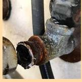
Corrosion caused one of the exterior faucets to break off the fixture.
